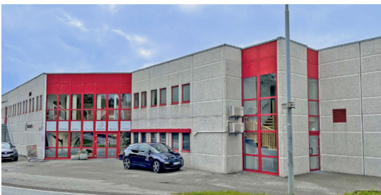
The stair builder has been using Compass Software since the early 1990s.
