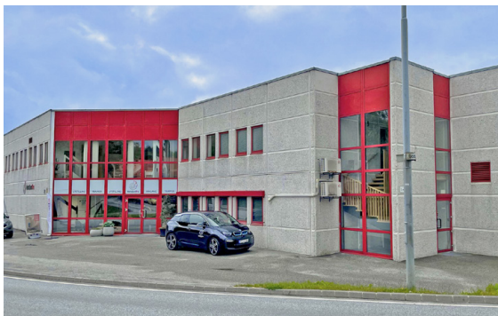
The stair builder has been using Compass Software since the early 1990s.
